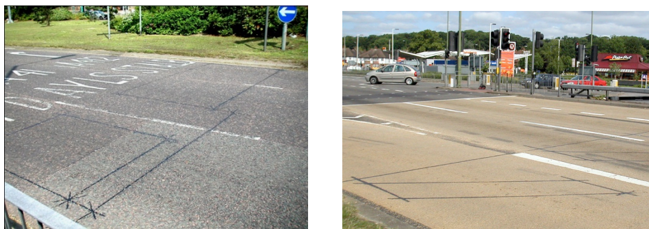
Figura 42 – Bucle inductive instalate in asfalt (exemplu)
